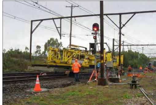
**(Above) A panel of point-work being moved into place.**
