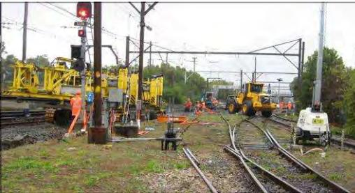
**(Above) Centre right is the de-commissioned “D” frame and lead. This section will be straight-railed from this point to the Ash Road connection.**
