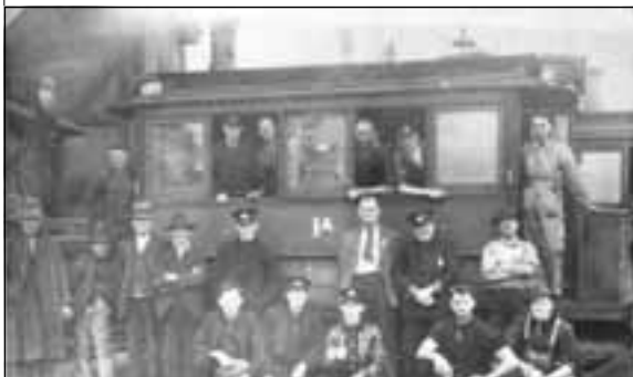
Motor IA photographed in 1937 at Kogarah depot. The number looks quite fresh and the end apron appears to be of the “round” type. Did a swap of motor bodies take place at this depot?
