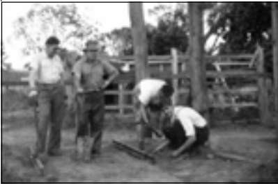
(Above & far Rt) At P’Matta Pk 1955. Contrast shed frames and first spike driving. In 1955 it was all 2nd hand poles, timber and sleepers. In 2007 it is steel frames, concrete sleepers and Pandrol clips.
