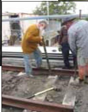
(Above & far Rt) At P’Matta Pk 1955. Contrast shed frames and first spike driving. In 1955 it was all 2nd hand poles, timber and sleepers. In 2007 it is steel frames, concrete sleepers and Pandrol clips.
