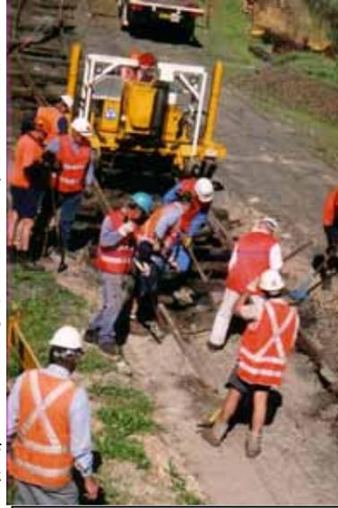
**The rail jack makes light work of lifting the aged track. Fortunately a hydraulic leak that materialized with the jack, came about at the end of the project. Volunteers from the museum and Rail Corp prise away old ballast.**
