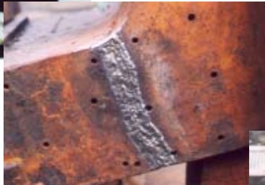
The weld on part of the yoke that forms the cylinders and smoke box end boiler support. The holes are from a previous repair done by the "Railways" in the form of a supporting plate.
