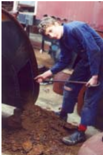
(left) Luke Tolhurst cleans out a mass of corrosion from the saddle tank.
