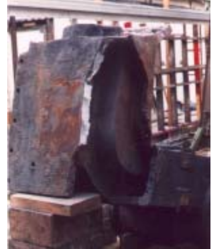
The cylinder prepared for the corner to be welded back on
