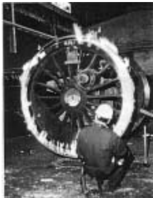
Letting people see how repairs are done in a safe environment. Some visitors are just as stimulated by this facet as by heritage train travel.
