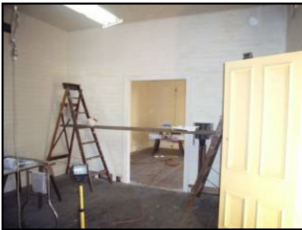
Above: Taken from room 2 looking into room 3. Painting is in progress.
