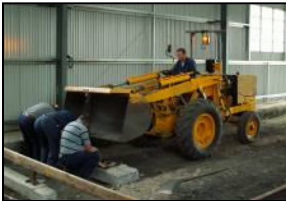
Above and Top Right: The Museum's newest (although far from new) piece of plant is put to good use in assisting with the laying of concrete sleepers inside the new Tram Shed. "Scoop" as it is more affectionately known, was obtained from Thirlmere and was in need of some major repairs before being employed in this work. Photos: Peter Butler.
