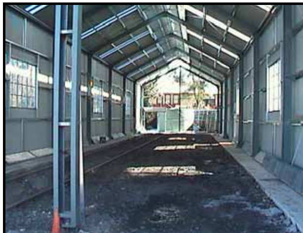
Above: The new STaRPS shed starts to take shape. These two views show frame work, and cladding on the southern wall. Below: Looking through the shed with cladding on both side walls and roof fitted. Note: Rails for the first siding in place. Photos: Ted Mullett.
