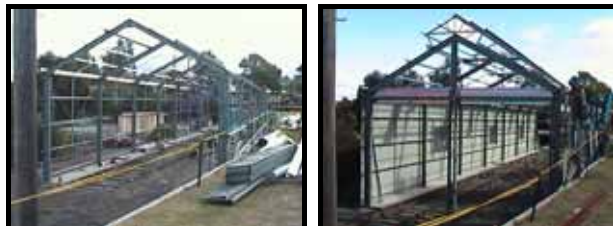
Above: The new STaRPS shed starts to take shape. These two views show frame work, and cladding on the southern wall. Below: Looking through the shed with cladding on both side walls and roof fitted. Note: Rails for the first siding in place. Photos: Ted Mullett.
