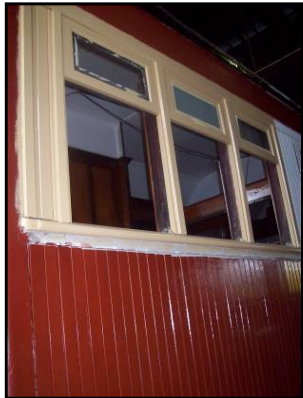
Above: Detailed photo of the match boarding and crown lights. Photo: Andrew Tester.
