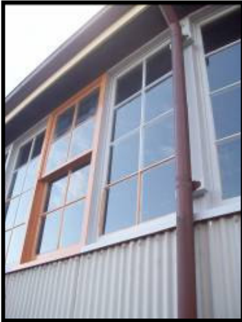
Left: Newly installed windows in Bay 7 receive their final coat of paint.
